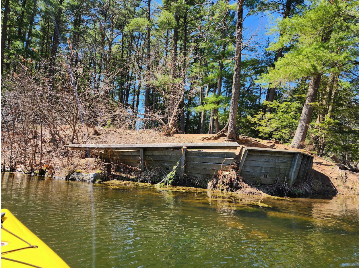
Area 3 East side (1 of 2 area 3's)
