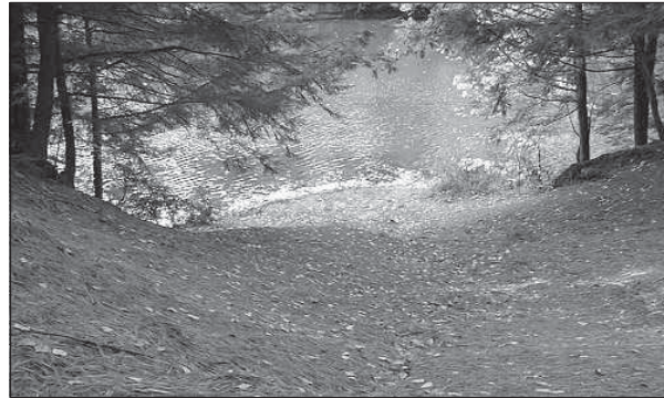
Pre-existing bank conditions at stabilization Area 2.
