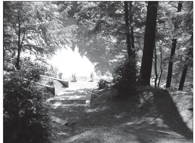
Bank Stabilization at the Westerly side of Area 3.
